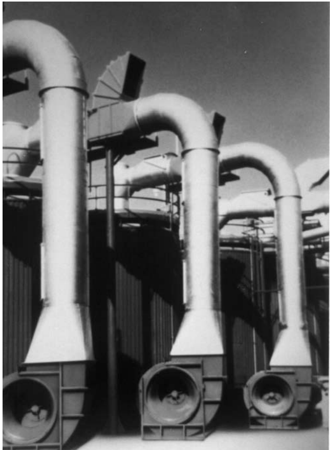
Figure 6. Well-designed duct configuration
